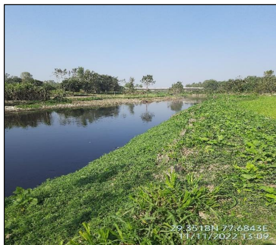
Figure 30 River Kali-West a/c Pur Baliyan village drain
