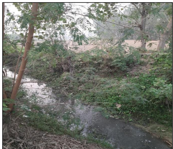
Figure 18 Titawi village drain
