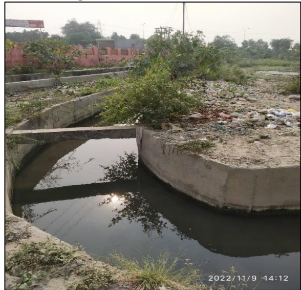
Figure 84 Hindon Vihar Right drain
