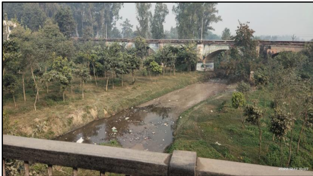
Figure 5 River Hindon at Janta Road Bridge, Saharanpur-Dehradun Marg
