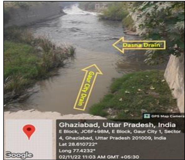
Figure 95 Dasna and Gaur city drain
