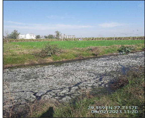
Figure 57 Deposition of sludge in Mansoorpur drain near National Highway-334
