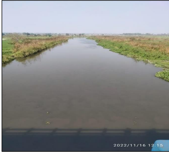
Figure 75 Hindon river downstream of Jawli drain
