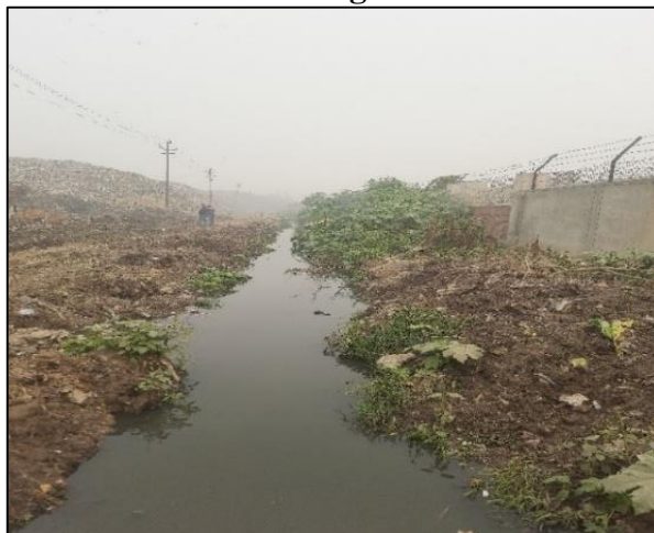
Figure 39 Nai Basti Khalapar drain (2nd order drain of Suzroo village drain)
