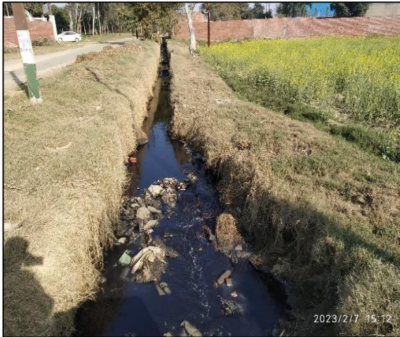
Figure 54 Begrajpur Industrial area drain
