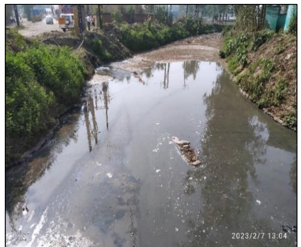
Figure 53 Sludge blanket formation observed in Dhandera drain at Jansath Road, Muzaffarnagar
